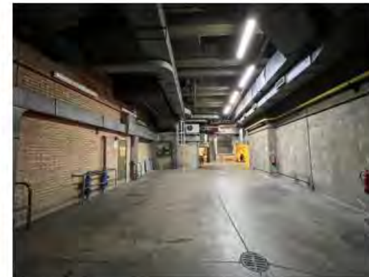
3 55 Old Broad Street service area
