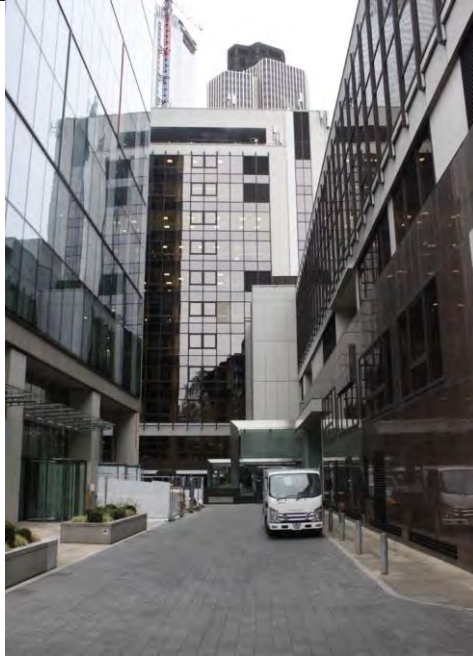
1 Spaces between buildings and approach to 55 Old Broad Street given vehicle priority
