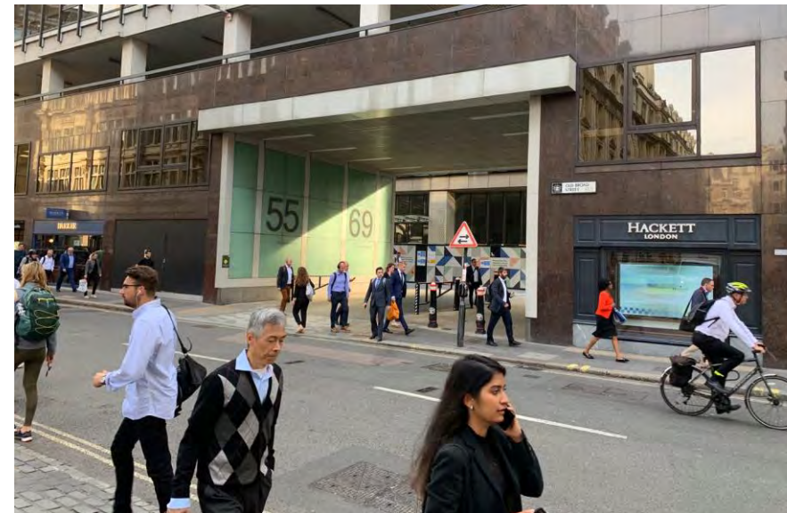
6 Old Broad Street: Old Broad St frontages very opaque and offer limited visibility to Dashwood and 55 Old Broad Street courtyard
