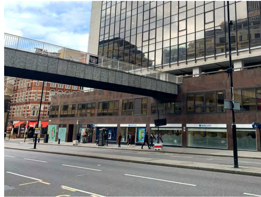
2 View from Wormwood Street: Hostile road with opaque and generally inactive frontages
