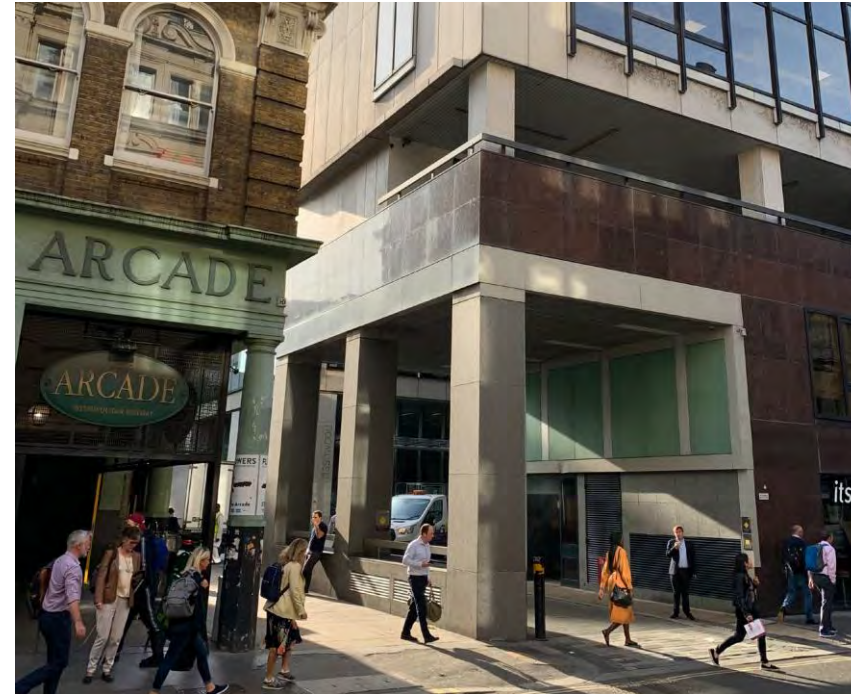
5 Approach to Site from north dominated by service road, fire escapes and plant ventilation
