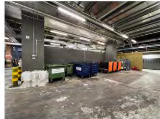
2 Service area shared between 55 Old Broad Street and Dashwood House
