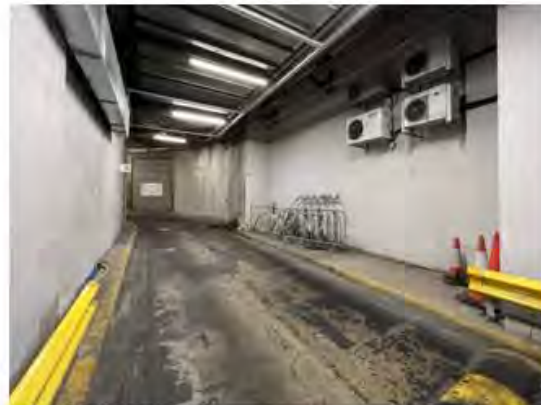
1 Ramp from ground level to Basement 2, shared between 55 Old Broad Street and Dashwood House
