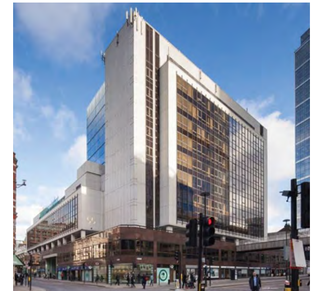
7 Wormwood Street/Old Broad Street Junction: Dark, opaque and underutilised frontages with difficult crossings and redundant bridge
