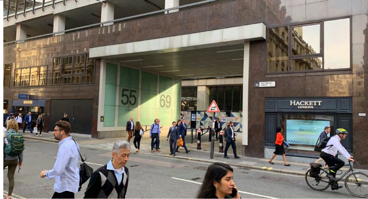
2 Entry to 55 Old Broad Street and Dashwood House concealed from Old Broad Street
